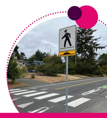
Raised crosswalks not only reduce vehicle speeds, but also provide accessibility benefits by allowing crossing to occur at sidewalk level.
