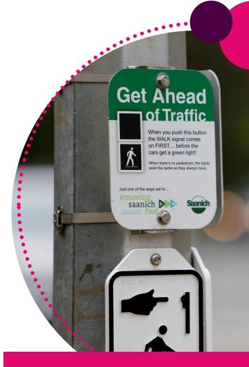
A leading pedestrian interval (LPI) gives pedestrians a head start when entering an intersection to enhance visibility and reinforce their right-of-way over turning vehicles
